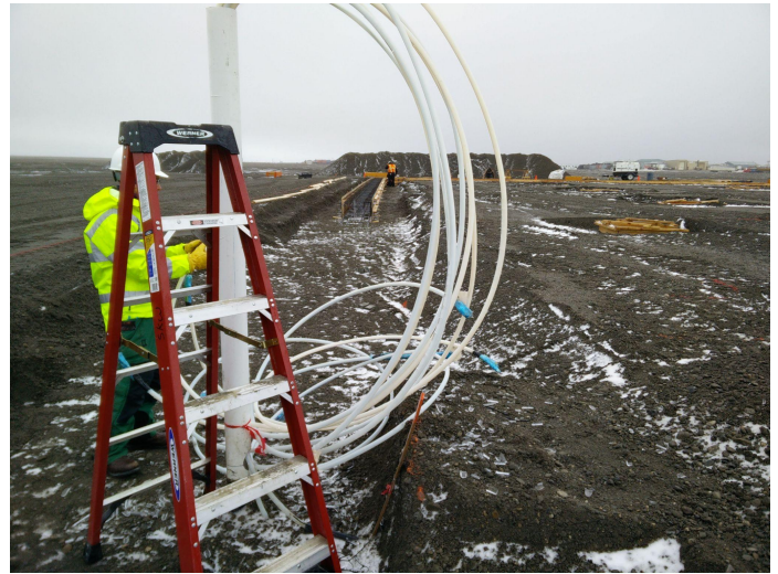
Cables encased in PEX were strategically installed to monitor ground layers, with vertical and horizontal DTCs reaching depths up to -202 ft (-61.6 m).
