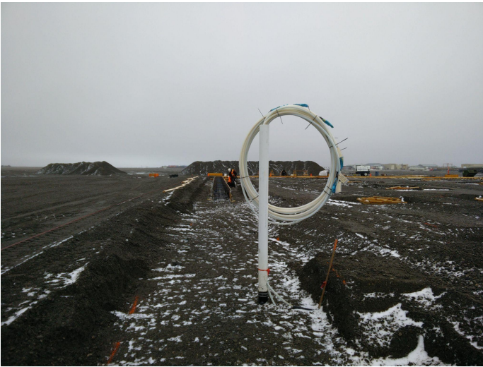
Cables encased in PEX were strategically installed to monitor ground layers, with vertical and horizontal DTCs reaching depths up to -202 ft (-61.6 m).
