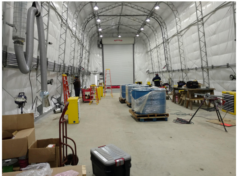
Interior of the truck offloading tent.
