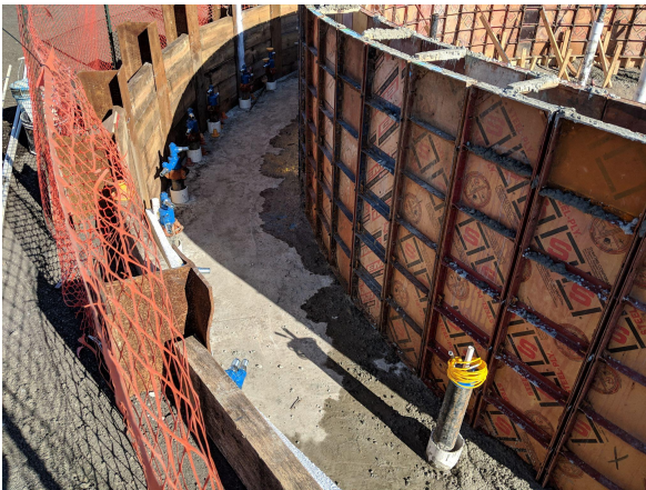
A Digital Temperature Cable within the frozen perimeter.
