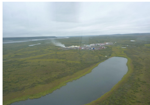
Aerial view of the National Petroleum Reserve, Alaska, captured from a helicopter during installation.
